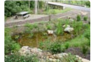
*Constructed wetlands used as a stormwater management control measure*
