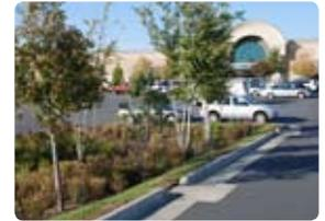
*An example of a bio-retention area in a mall parking lot in Charlotte, NC. The curb cuts allow stormwater to enter the retention area.*
