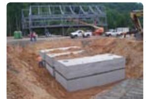
*Cistern to store 60,000 gallons of rainwater for irrigation and toilet flushing at a new school being built by the Eastern Band of the Cherokee Indians*
